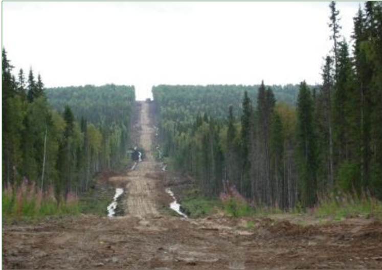
2009 road construction in Karpogory forest district
