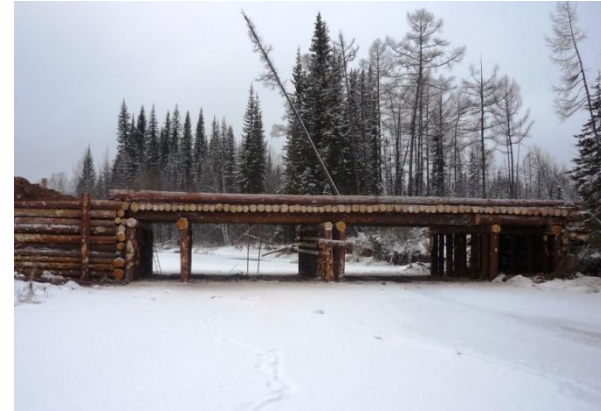
RusForests responsibility in development of internal roads and bridges in the new leases
