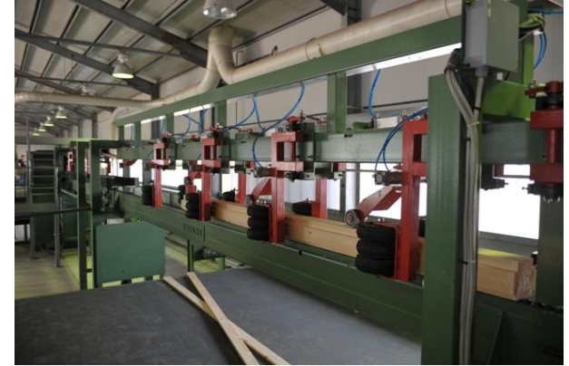
First two side boards separated from the cant upon exit from the first machine
